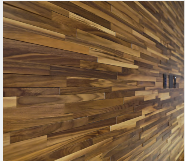
Toyota also emphasizes recycling through materials choices. This wall in the lobby of our new R&D campus in York, Michigan, is constructed of scrap pieces of wood, expertly combined and finished to create a unique look.
